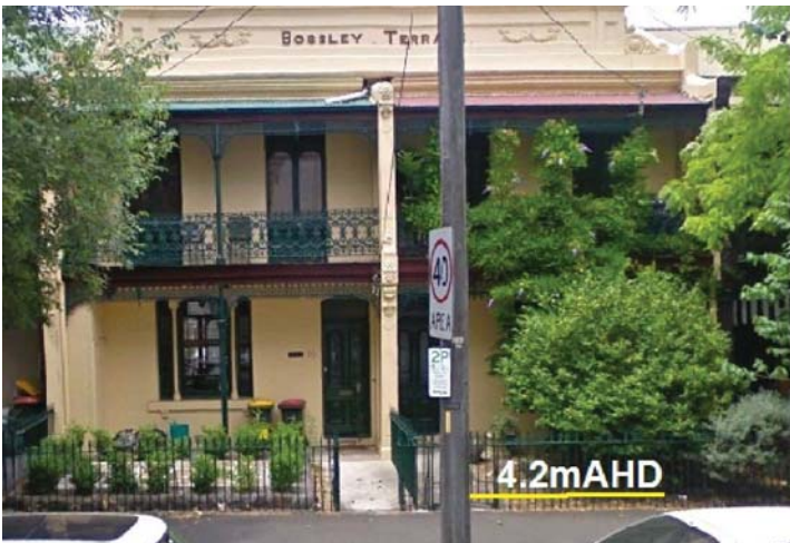
Approximate elevation of regular flooding along front fence near Crown Street Low Point. 4.2m AHD
