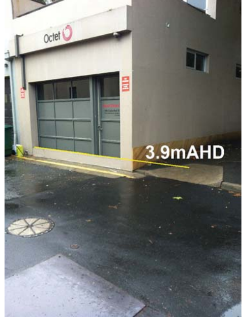
Flood barrier installed at Bossley Terrace, with approximate elevation of barrier height. 3.9m AHD
