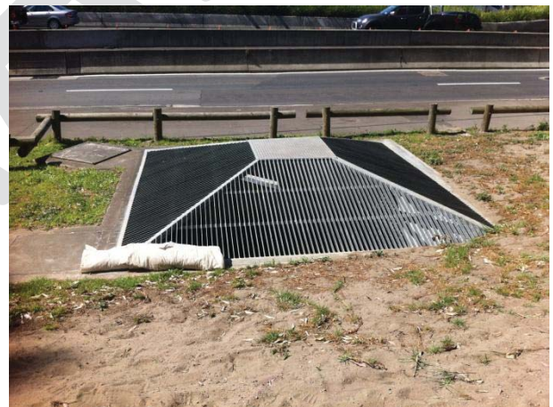
Photo 16: 4 m by 4 m inlet pit
