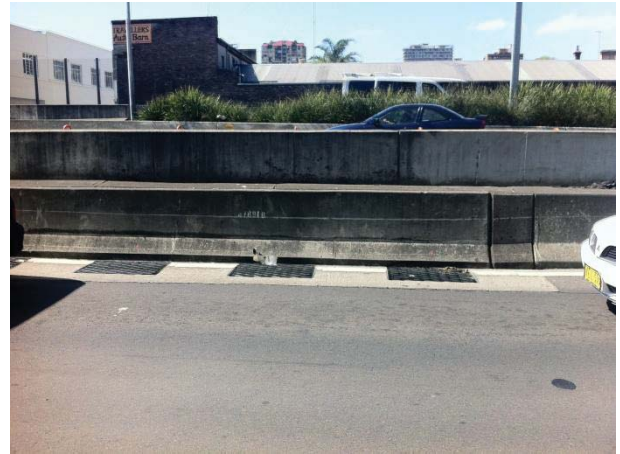
Photo 18: 4x0.6x1.0 m grated inlets
