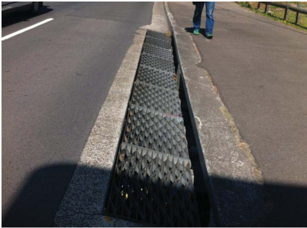
Photo 17: 7.2m lintel and 7x0.6x1.0 m grated inlets
