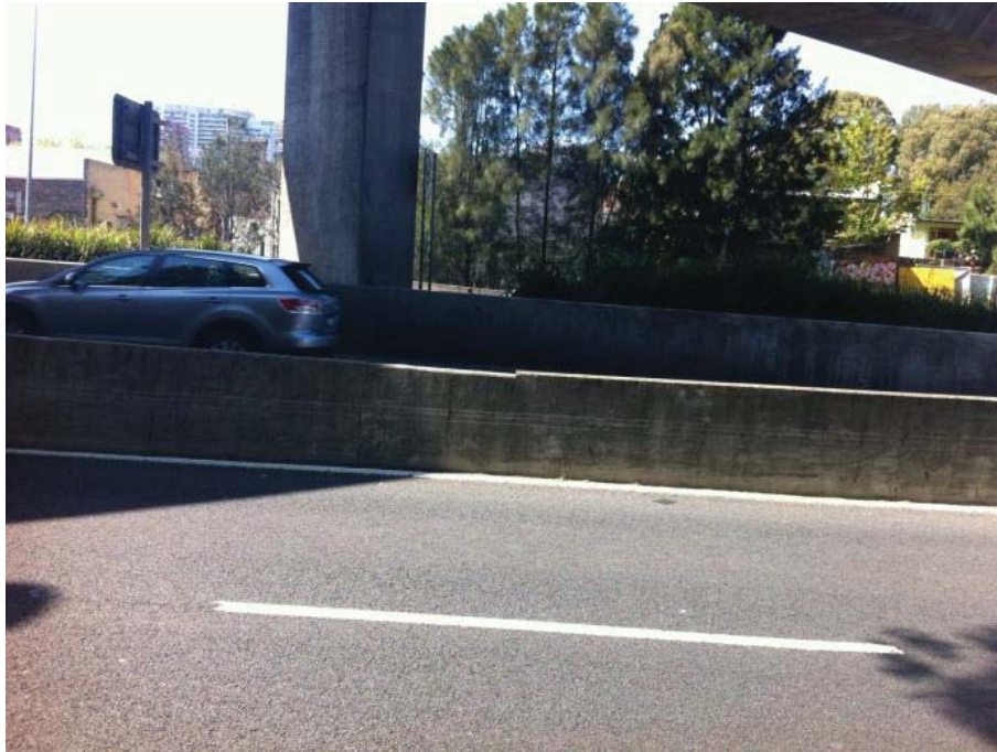
Photo 11: Divider between Palmer Street and the Eastern Distributor
