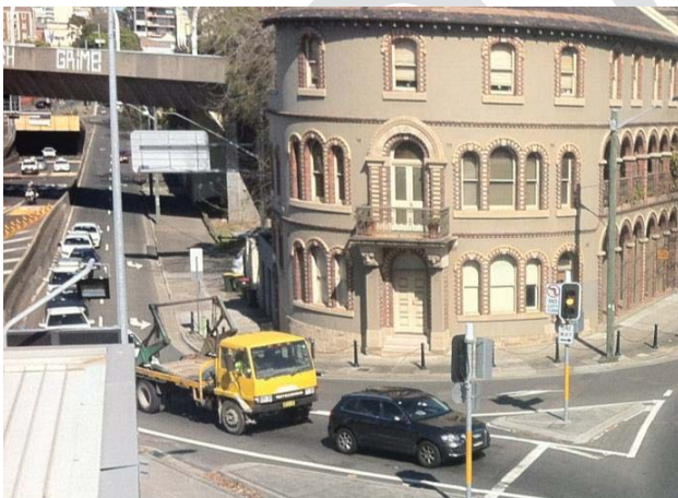
Photo 15: Palmer Street Low Point
